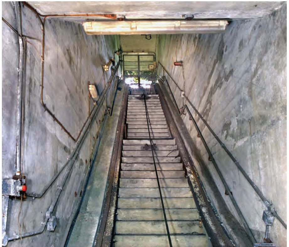
A final steep flight of stairs took us up to the surface and out through the emergency exit. Note the trolley rails either side of the steps and the winch cable in the centre of the steps.
